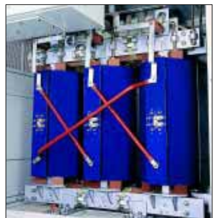
Cast Resin Transformer
