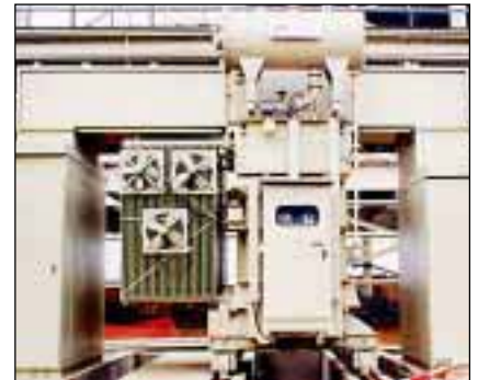
20 MVA, 33/11 kV Power Transformer with PDO, Oman
